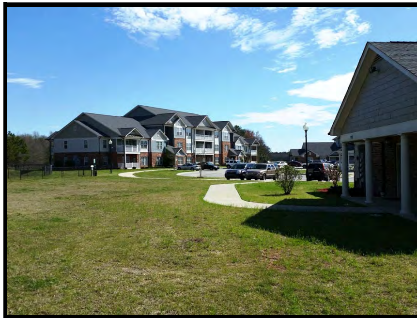
East view from site
