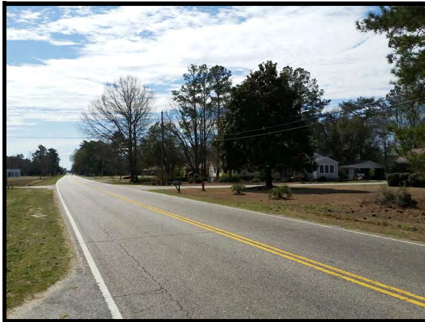
Streetscape south view of South 4th Street
